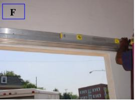
Slide panels #2 and #3 to the right hand side of track-The track that does not have the operator
